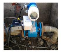
The measured liquid must be conductivity liquid of serosity of which the conductivity should be more than 50 s/cm the medium should not contain much magnetic matter of air bubbles. Pressure grade lining material, electrode material and structure type should be selected according to the medium's temperature corrosiveness, abrasion, etc. Normally the sized of flow meter should be the same as the pipe diameter.
